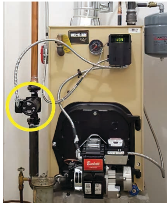
Figure 13-20: Circulator located on return line
