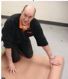
Figure 3-16: Cover work areas
