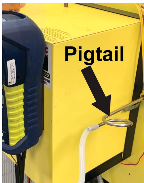
Figure 7-16: When taking over fire measurements with an analyzer, the use of a small diameter steel pipe with attached flexible tube, commonly referred to as a pigtail, will protect probe from extreme temperatures.
