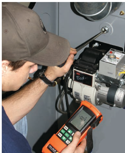
Figure 7-7: Over-fire draft measurement
