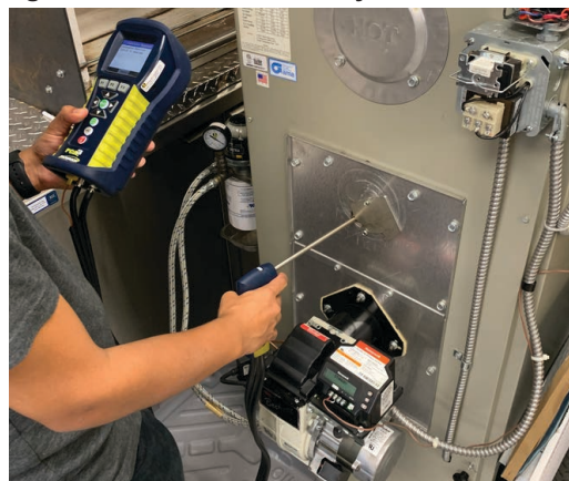
Checking draft over the fire
