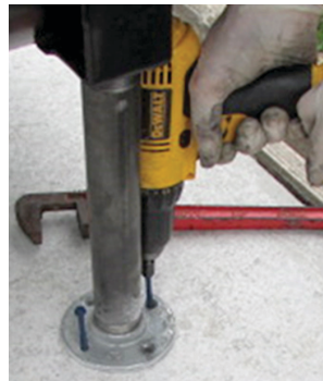
Fig 6. Concrete screws installed after hole has been cleaned and adhesive added
