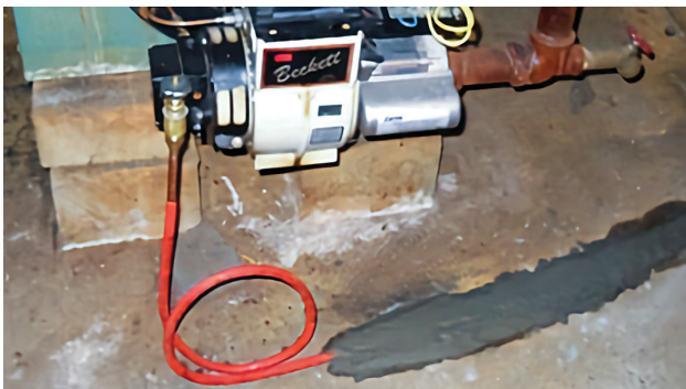
All fuel lines that contact concrete or soil should be protected in a continuous run of corrosion resistant tubing.
