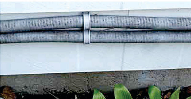
As shown here, fuel lines should be reasonably protected from damage and secured.
