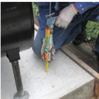
Fig. 4. Adding adhesive to the drilled hole
