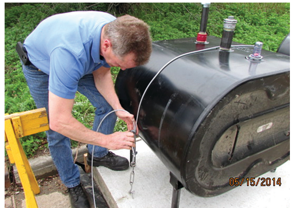
Fig. 13. Installer performing wire rope tie-down.
