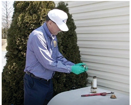
Be sure to remove the vent cap to make sure a screen is in place!
