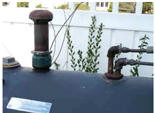
Top draw line should be insulated on outdoor installation.
